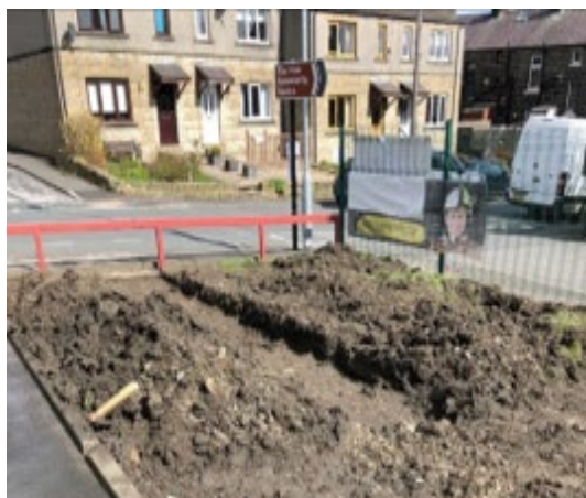
Picture taken during the garden renovation
